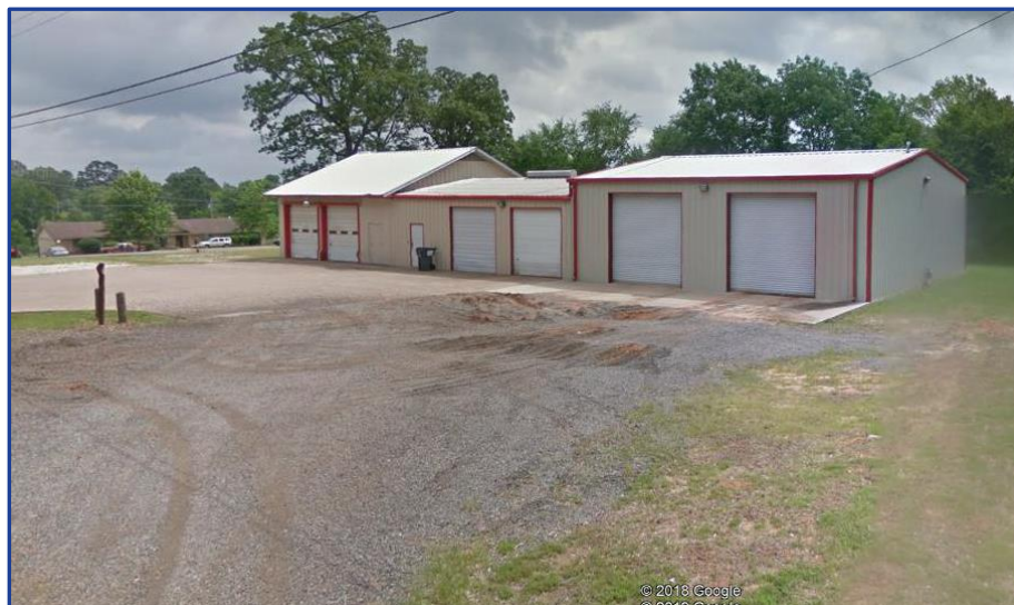
Figure 37: Jackson Heights Station 1 Driveway and Apparatus Pad
